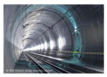
Stainless steel cable channels carry wiring and support composite escape handrails in the Gotthard Base Tunnel.
